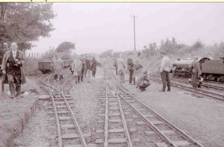
(Above) Two shots in R&ER Beckfoot Quarry in 1954, showing a single bladed point and a 3-way point with rake of stone wagons. (Below left) a 1966 shot at Ravenglass where I strongly suspect that the 3-way point had found a new use in the carriage sidings. (Below right) R&ER Sankey Barrow card purchased early 1950s River lrt on mixed gauge south west of Murthwaite
